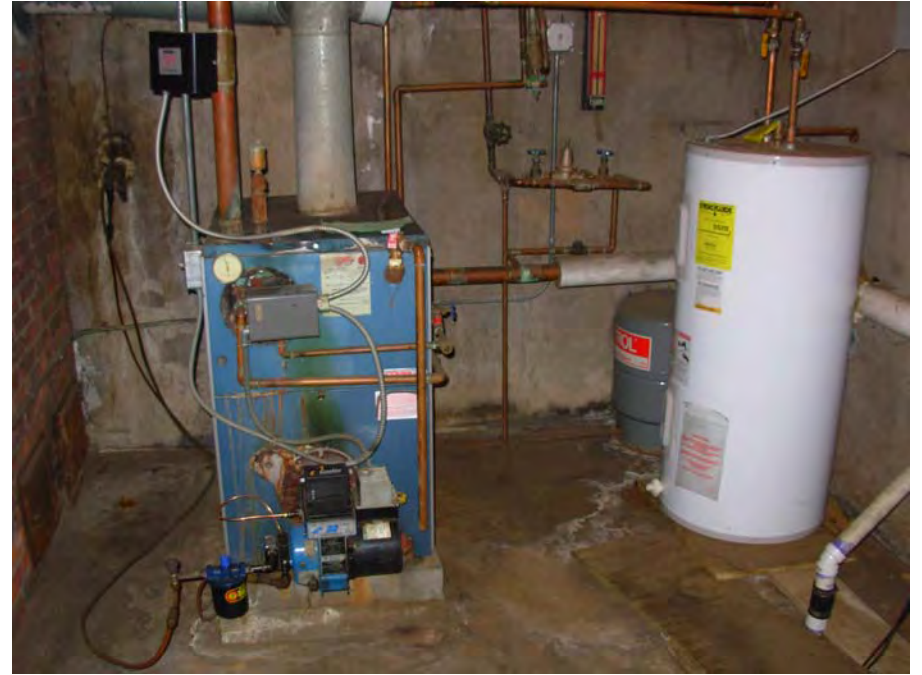
10. Heating and DHW equipment serving admin.-cmnty. building
