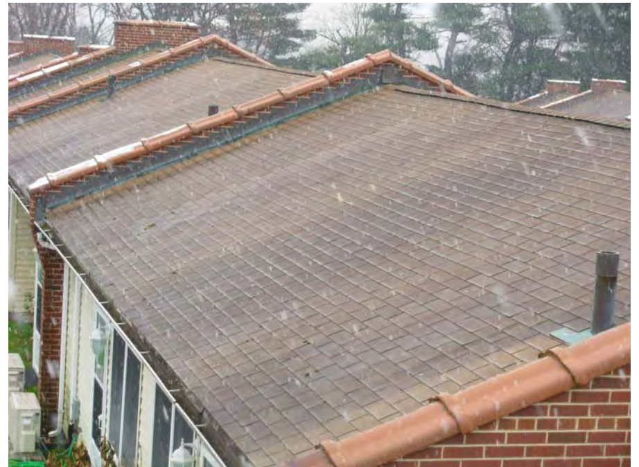
4. Roofing shingles display staining and organic material growth
