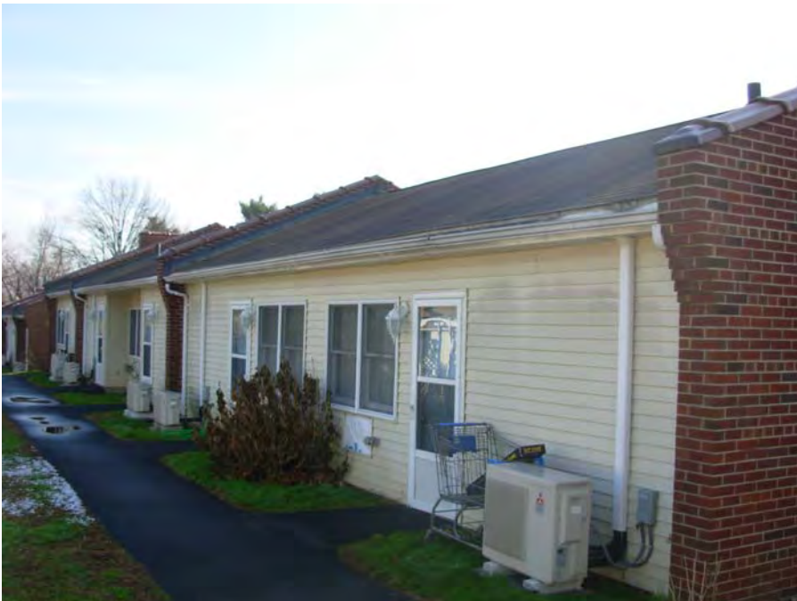
3. Building exteriors to have vinyl siding, windows, doors replaced
