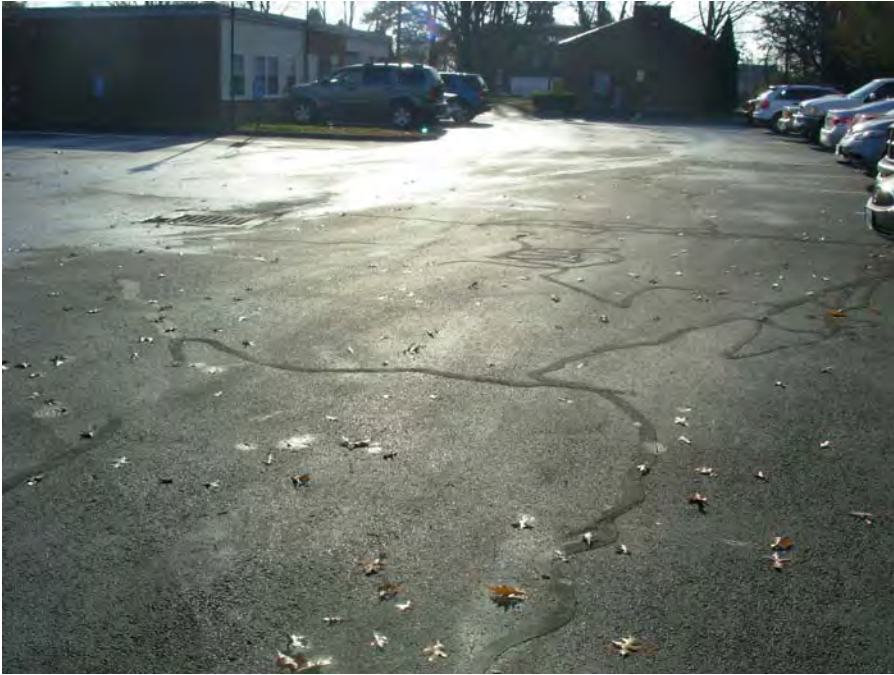
1. Parking and walkway surfaces recently crackfilled and sealcoated
